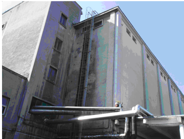
Fig. 2. General view of the cold store in Włocławek
